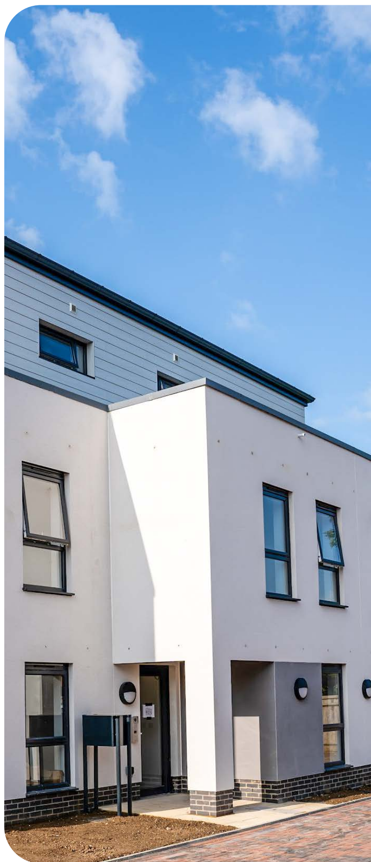
Crofts Court, affordable homes in Oxford.
