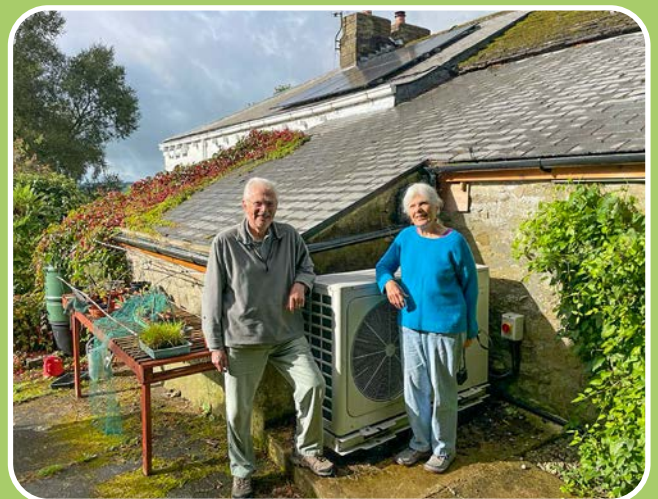
Savings Members Daniel Powell and Lindy Williams with their new heat pump and solar panels.
